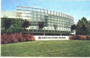
The CHM building
